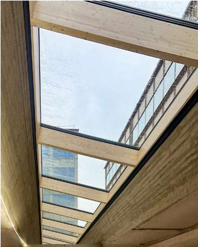
Installed HUF elements for the Textiltorget project.
