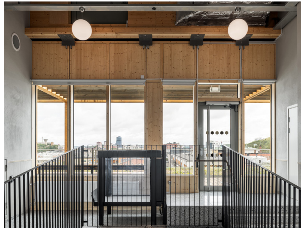
Interior view of Textiltorget's completed HUF installation, showcasing exposed glulam timber framing and floor-to-ceiling glazing.
